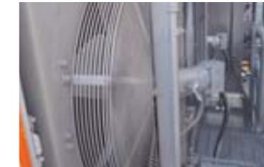
Four oil coolers are used for optimal cooling efficiency. They are positioned far from the engine radiator for even better cooling potential.
