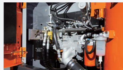
Grouped remote filters and inspection points
